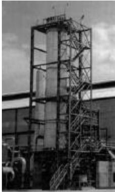
An ammonia converter 23 meters high installed at the Aonla plant in India by Haldor Topsøe. From *Enriching the Earth*.
